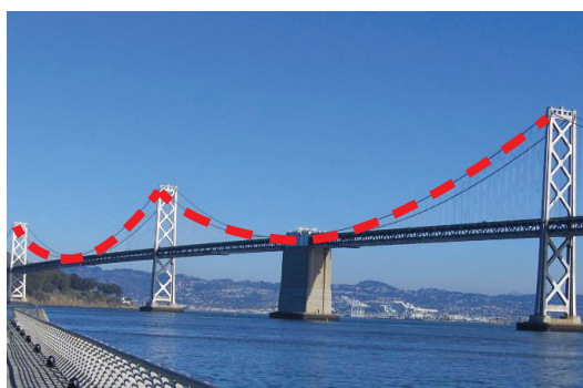
Oakland Bay Bridge in California with cables following a parabolic curve
